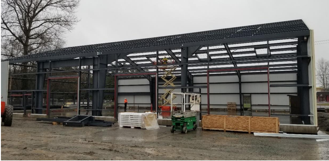
Installation of Structural Steel Supports for Technology & Storage Building
