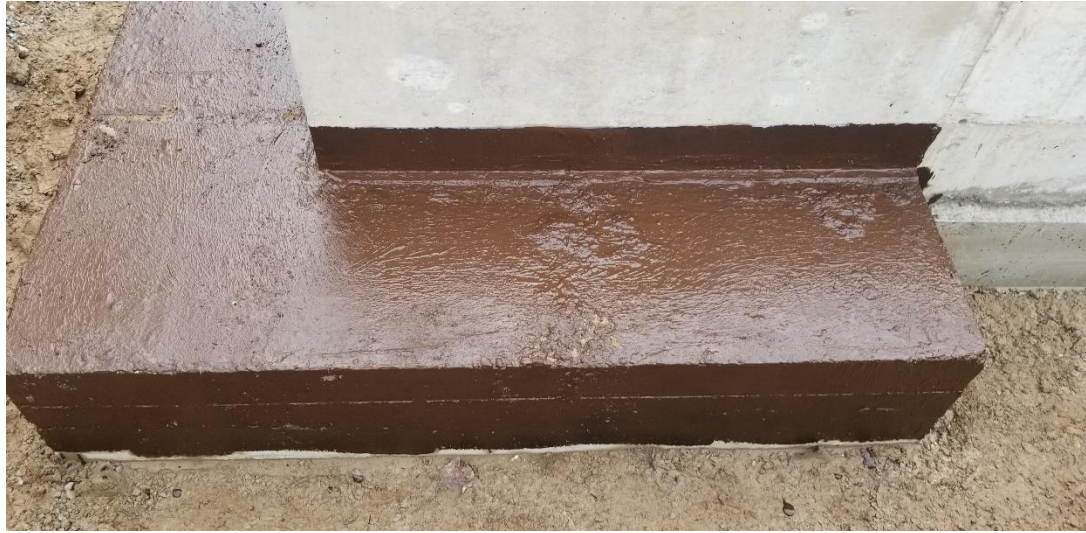
Dampproofing at Concrete Foundations
