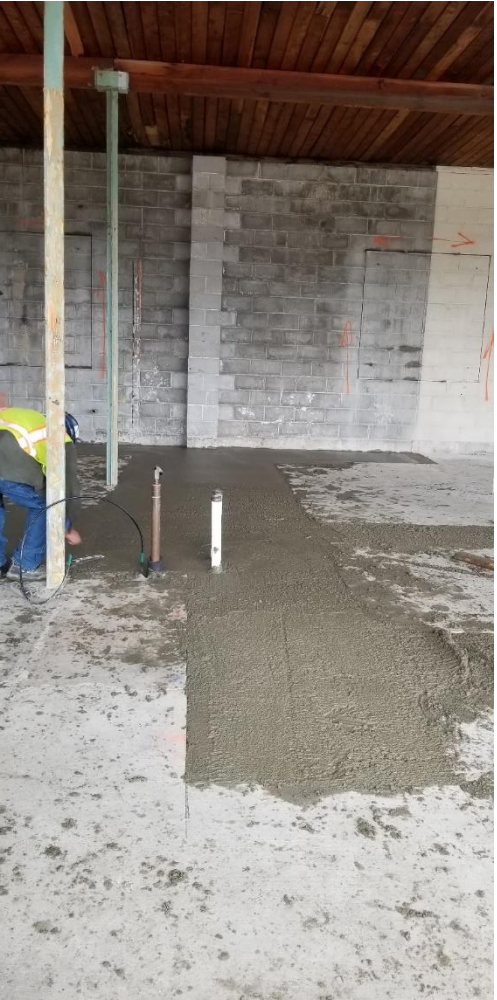
Concrete Foundation and Slab Pourback
