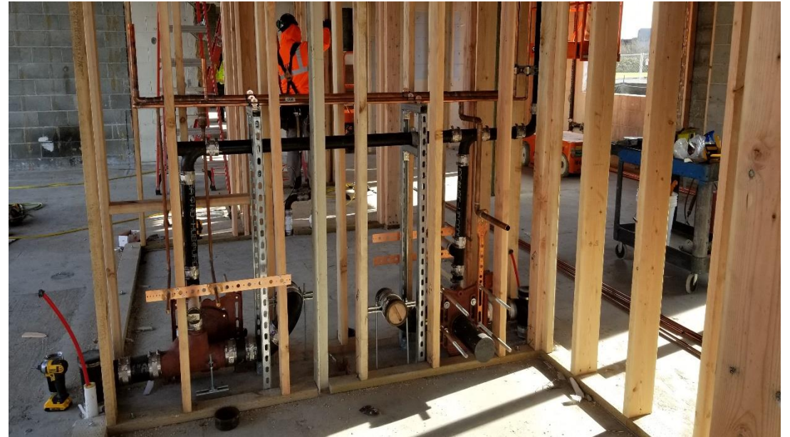
MTC Restroom Plumbing Rough-in
