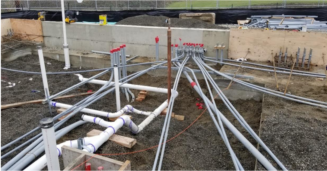
Underslab Plumbing and Electrical for Technology & Storage Building
