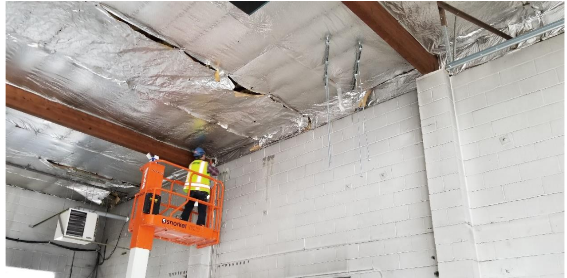
HVAC Equipment Support Installation
