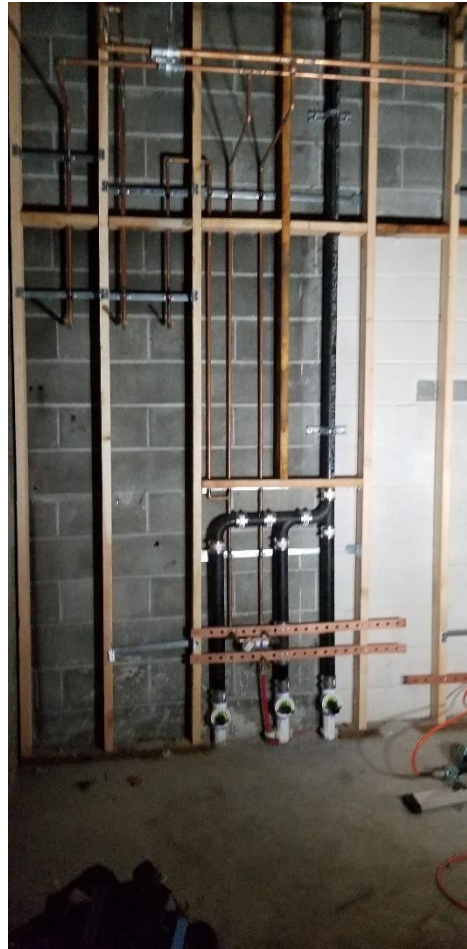
Shop Restroom Plumbing Rough-in and Framing
