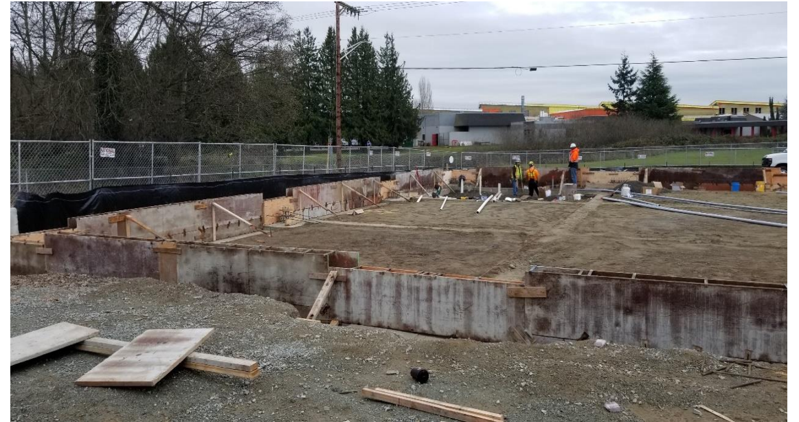
Foundation Wall Formwork
