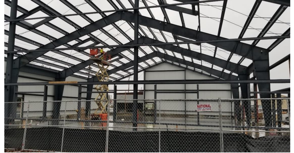
Installation of Structural Steel Supports for Technology & Storage Building
