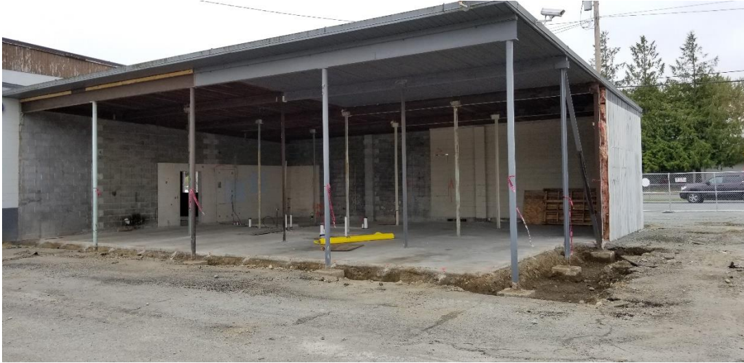
Subgrade Prep for New Footing and Foundations
