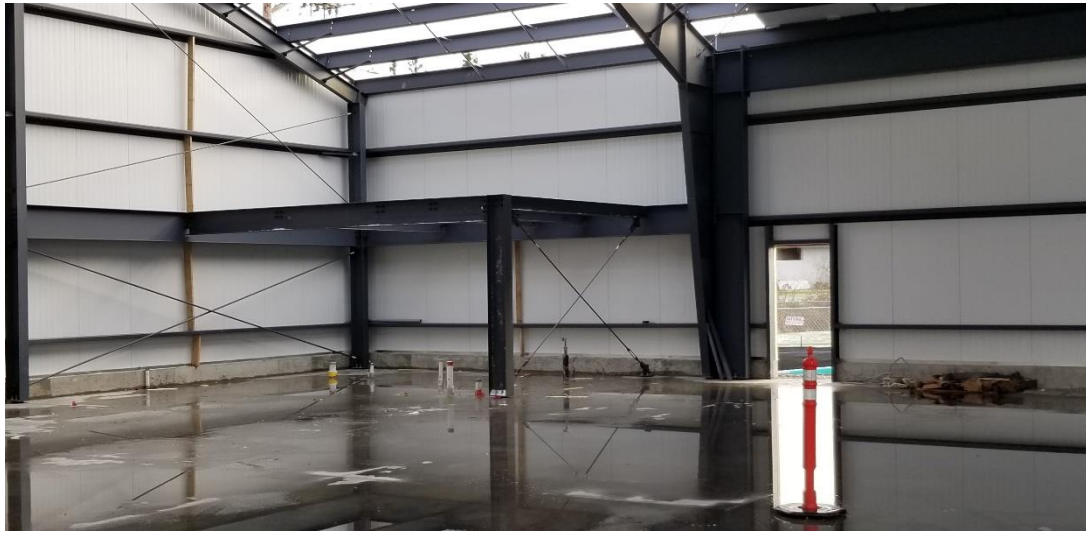
Platform for Mechanical Room
