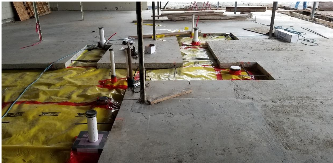
Vapor Barrier Under New Concrete Slab
