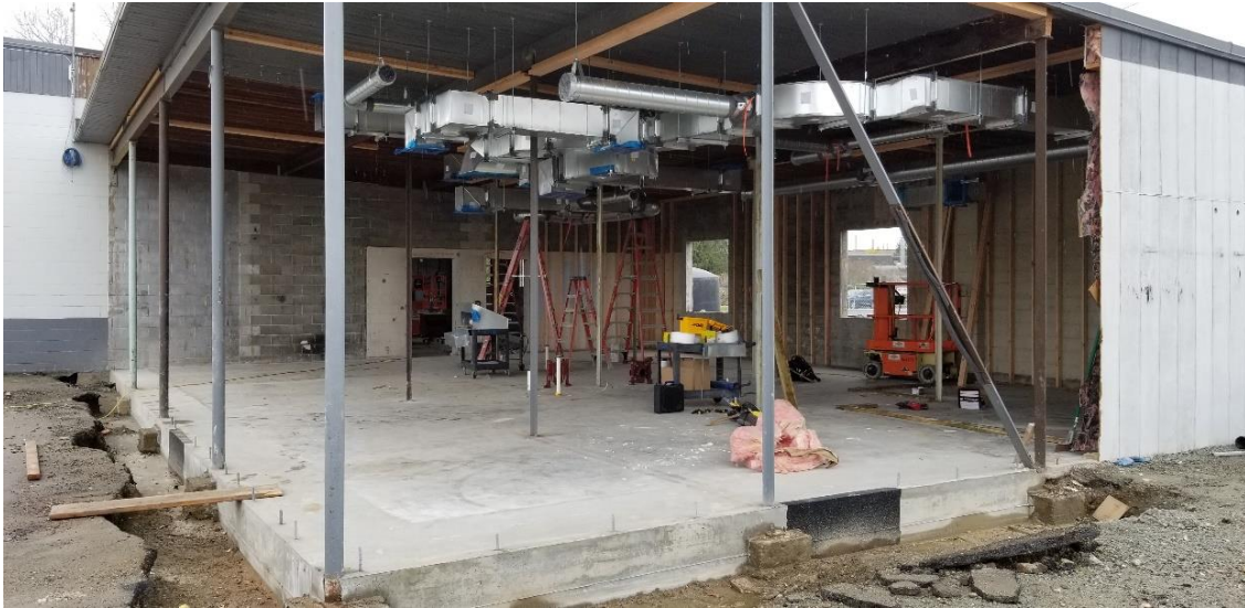
HVAC Ductwork Installation
