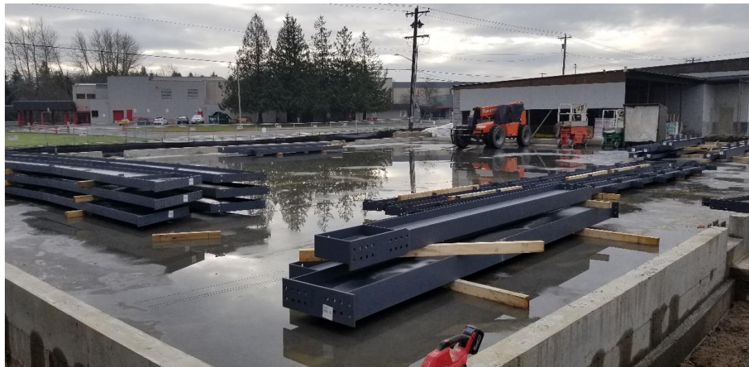
Structural Steel Columns for Technology & Storage Building
