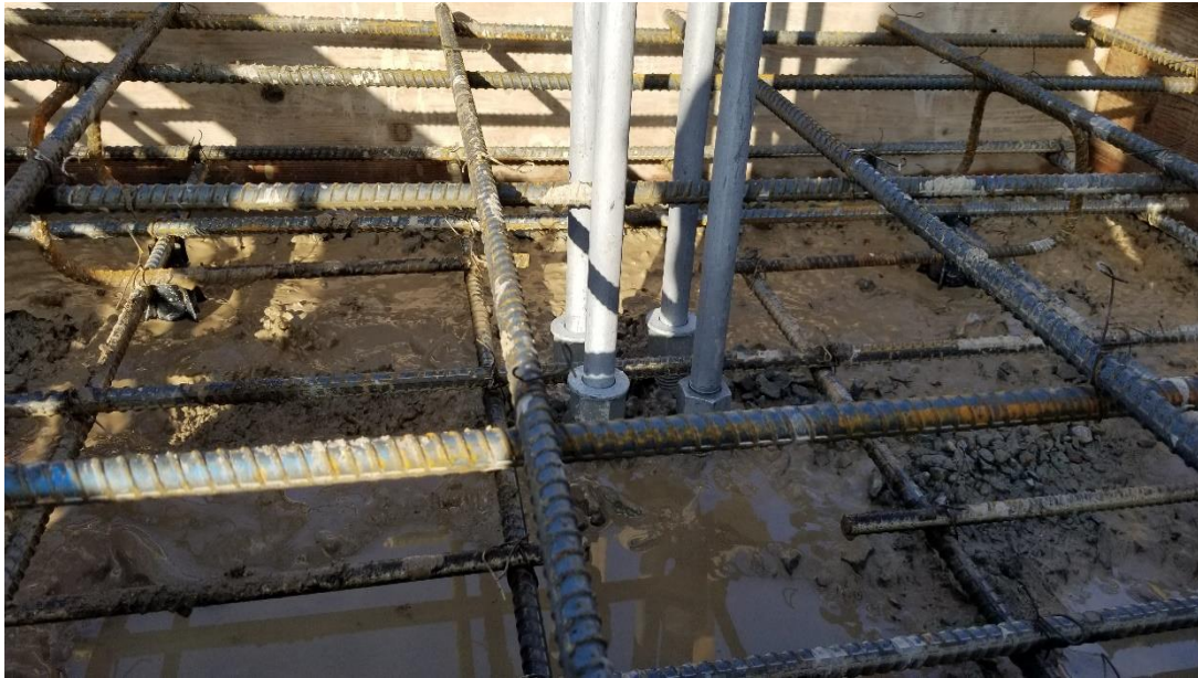
Reinforcing Steel and Structural Imbeds at Column Footings
