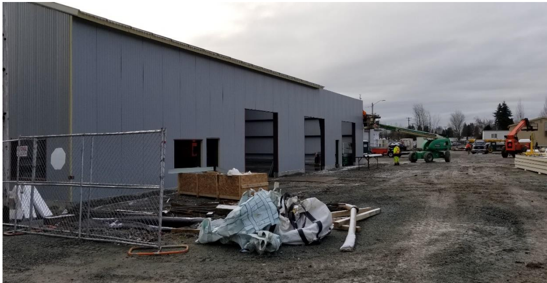
Installation of Insulated Wall & Ceiling Panels for Technology & Storage Building
