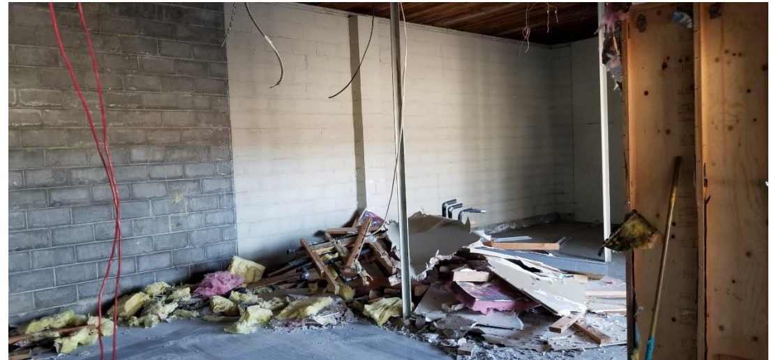
Demolition of the MTC
