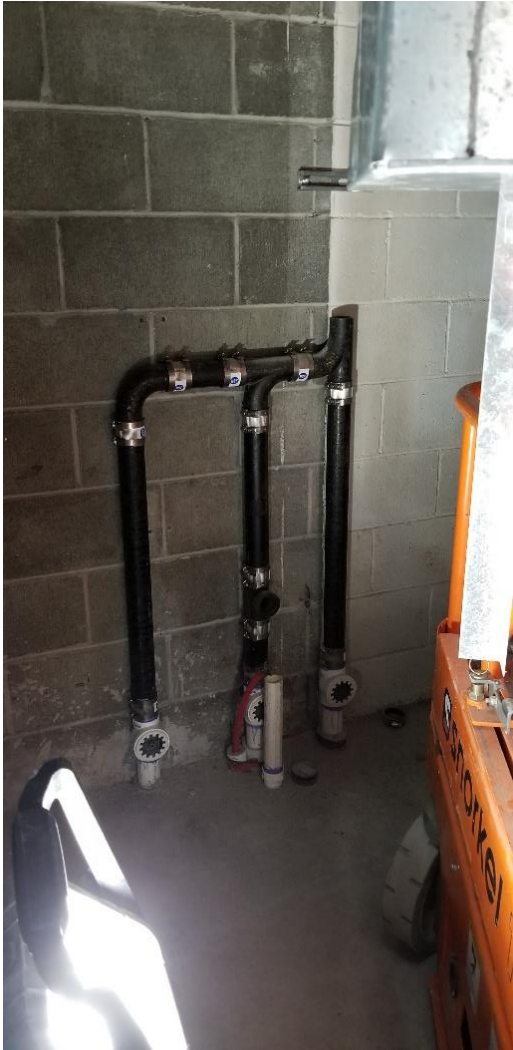
Shop Restroom Plumbing Rough-in and Framing
