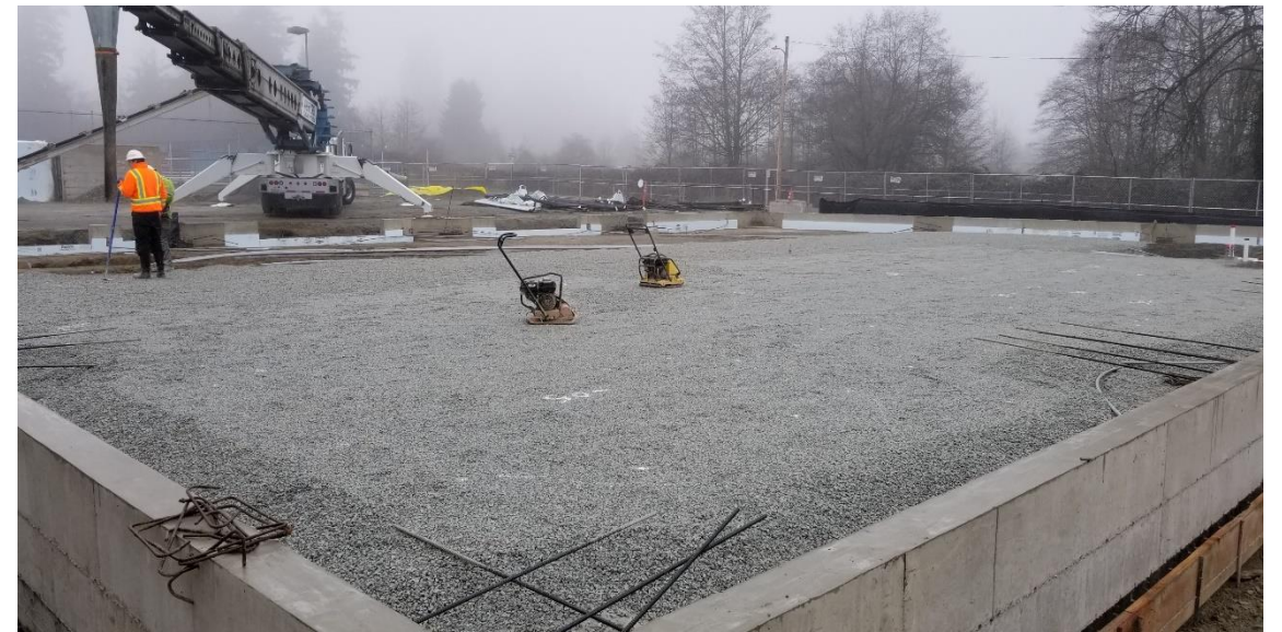
Underslab Gravel Subbase
