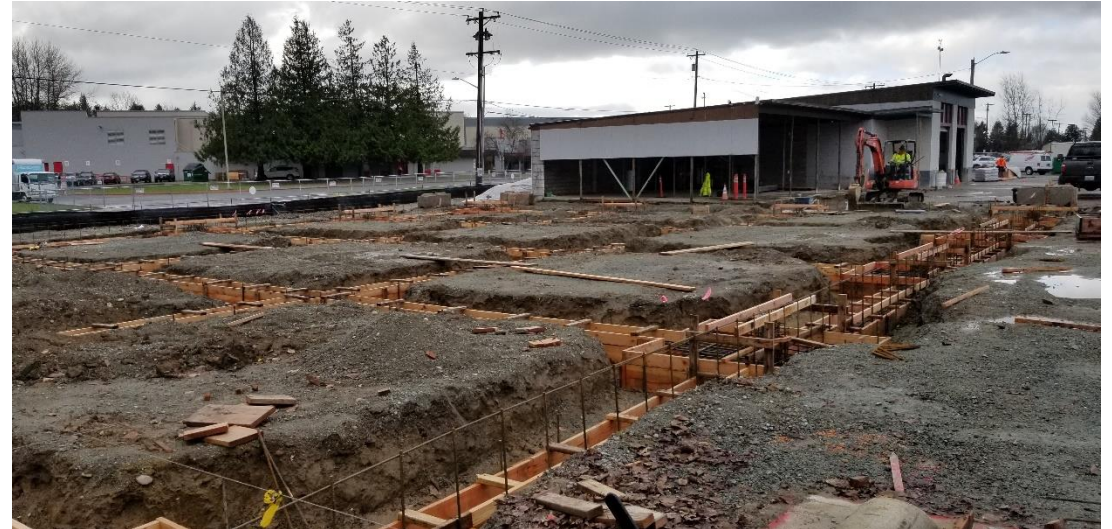
Footings Formwork for New Technology & Storage Building
