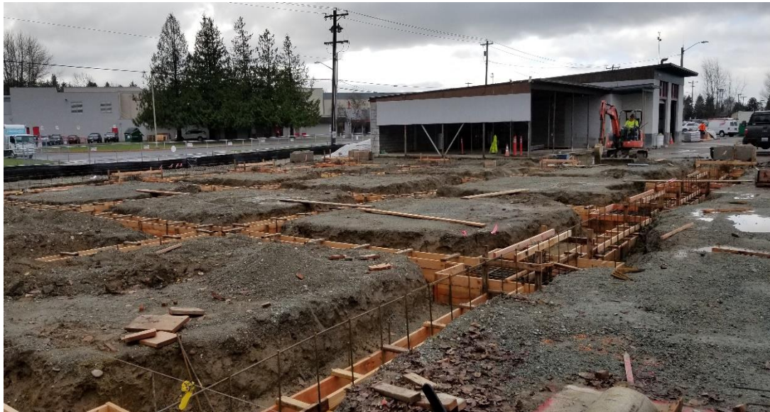
Footing Formwork for New Technology & Storage Building
