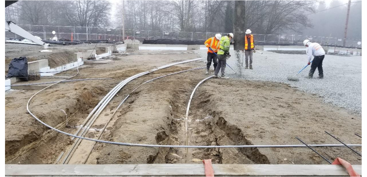
Underslab Plumbing and Electrical for Technology & Storage Building
