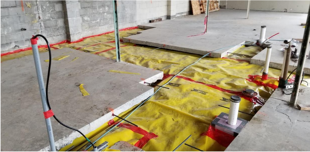
Slab on Grade Prep around Under Slab Plumbing Rough-in
