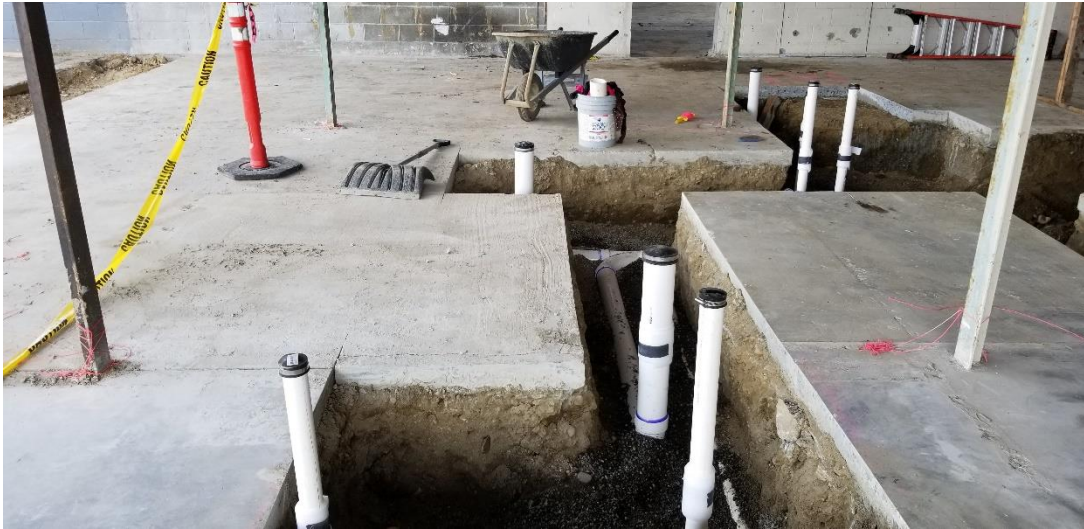
Under-slab Plumbing Rough-in
