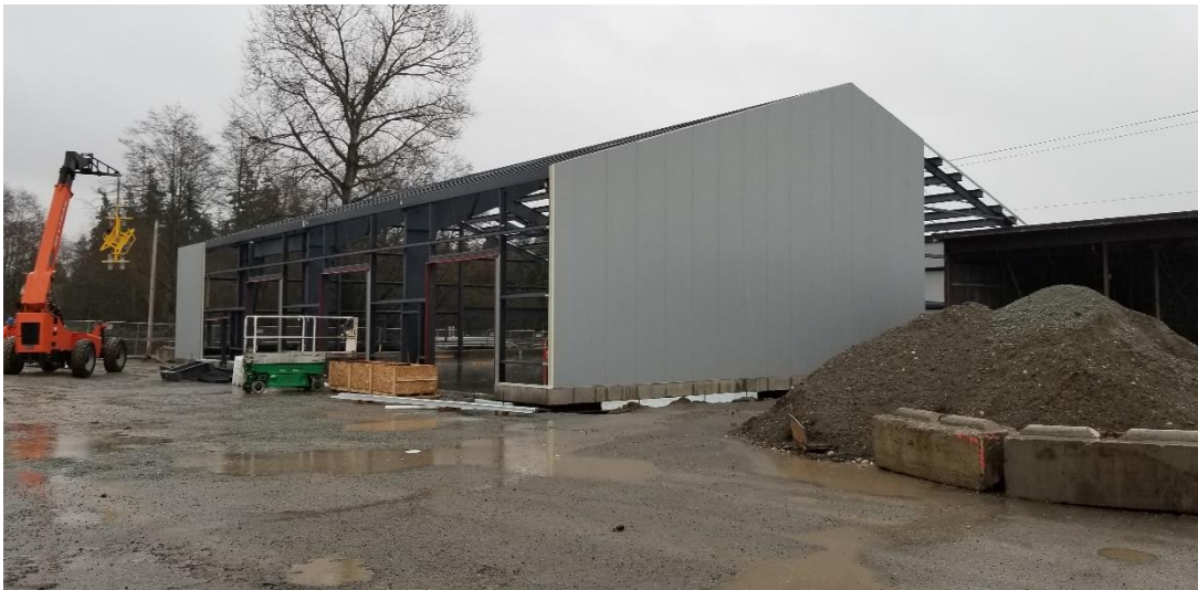
Installation of Insulated Wall Panels for Technology & Storage Building
