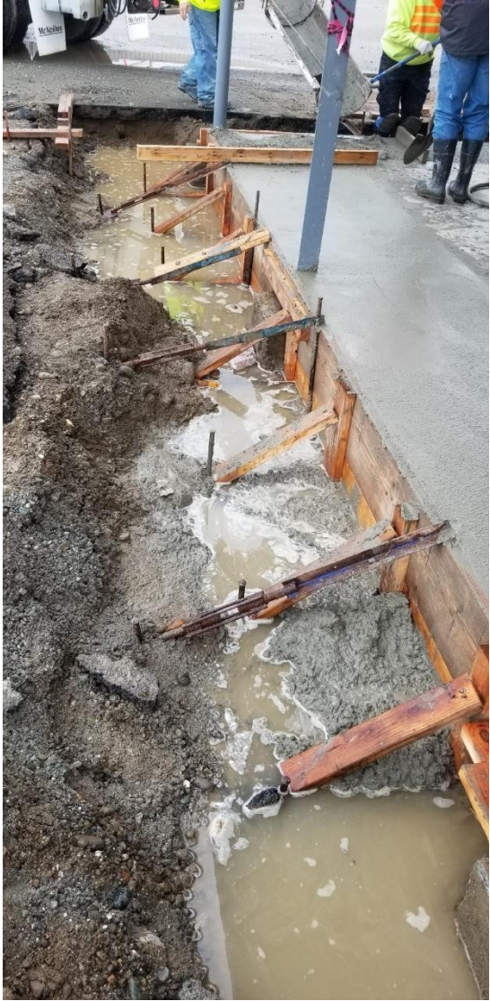
Concrete Foundation and Slab Pourback
