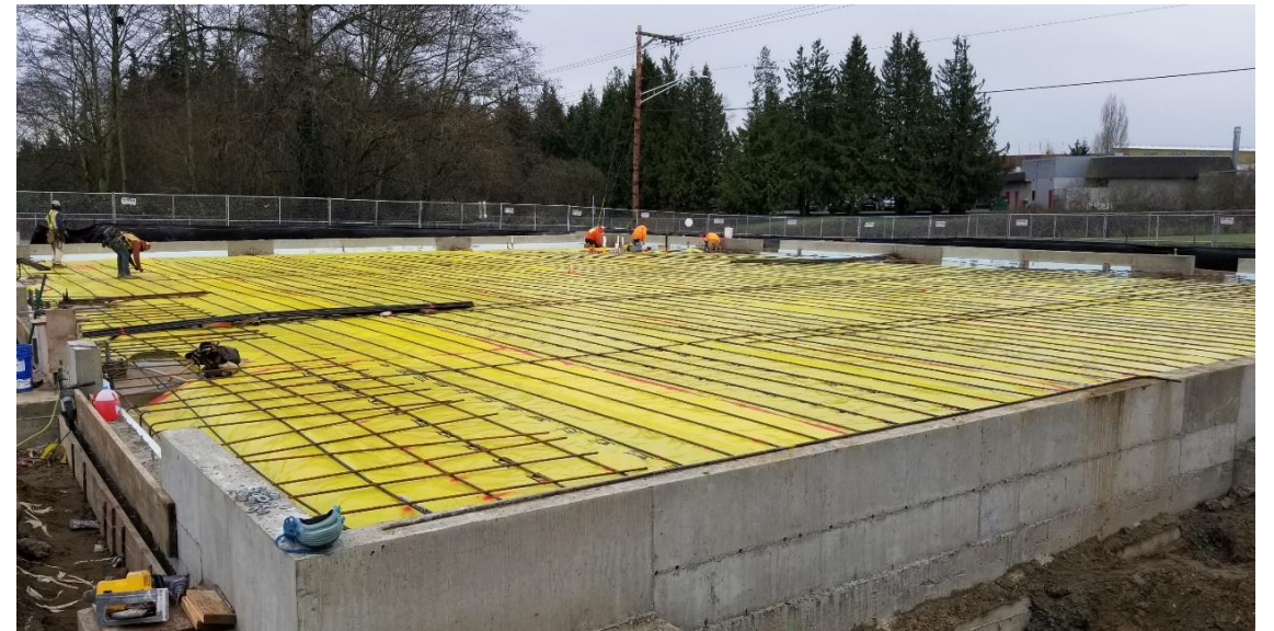
Vapor Barrier and Reinforcing Steel Under Concrete Slab
