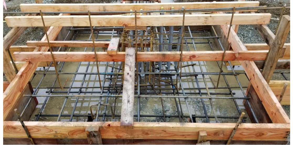
Reinforcing Steel at Column Footings
