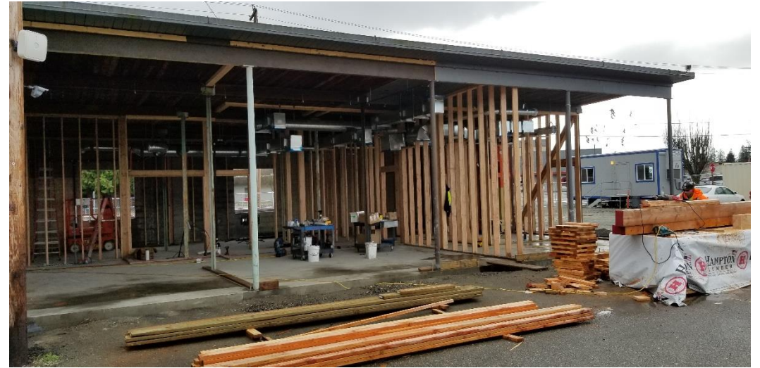
Framing for Administration Offices
