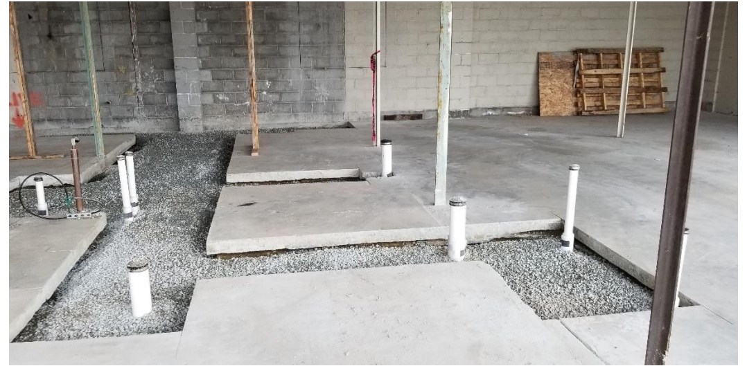
Under-slab Plumbing Rough-in
