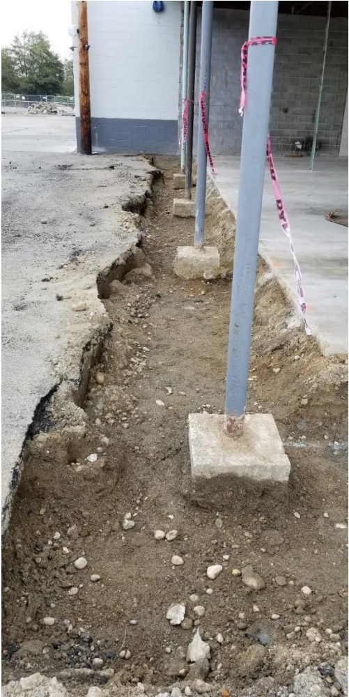
Excavation for Foundations
