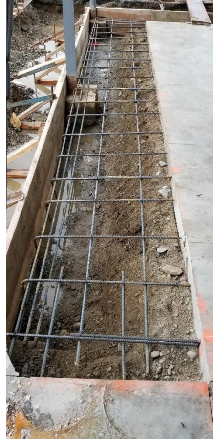
Excavation and Reinforcing Steel & Formwork for Footings and Foundations
