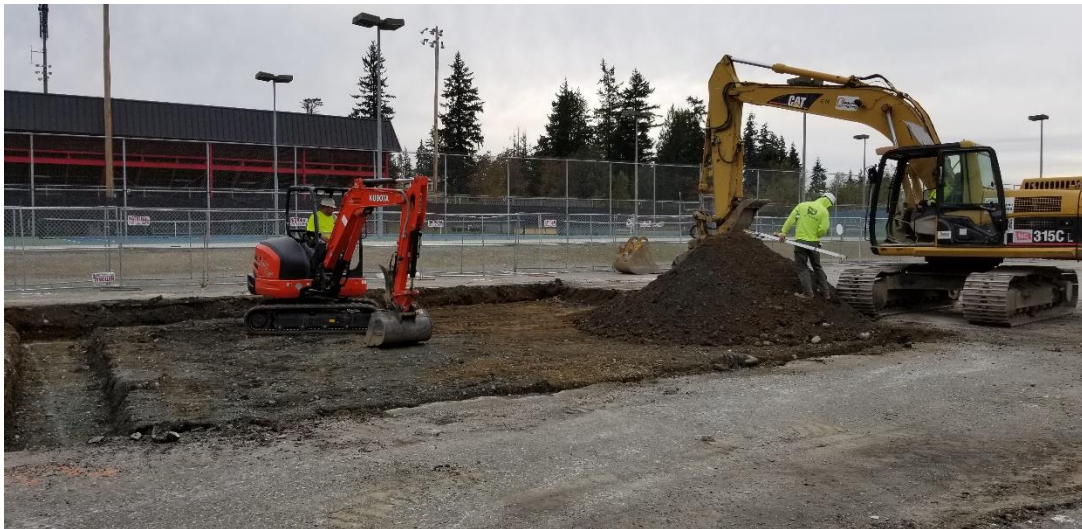
Subgrade Prep for Portable
