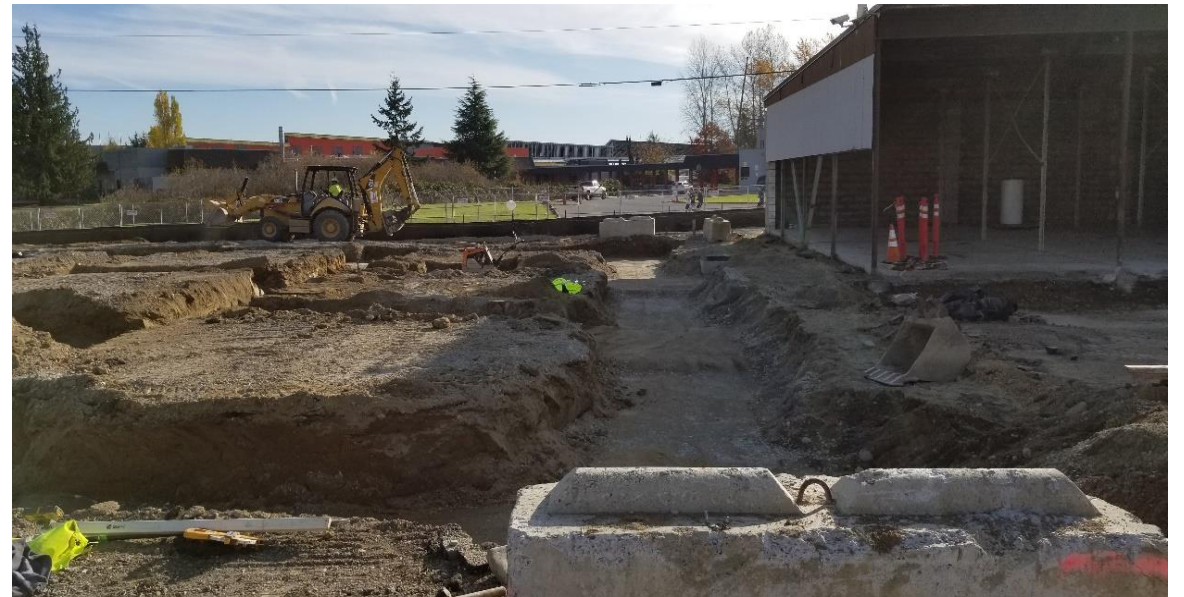
Footing and Foundation Excavation
