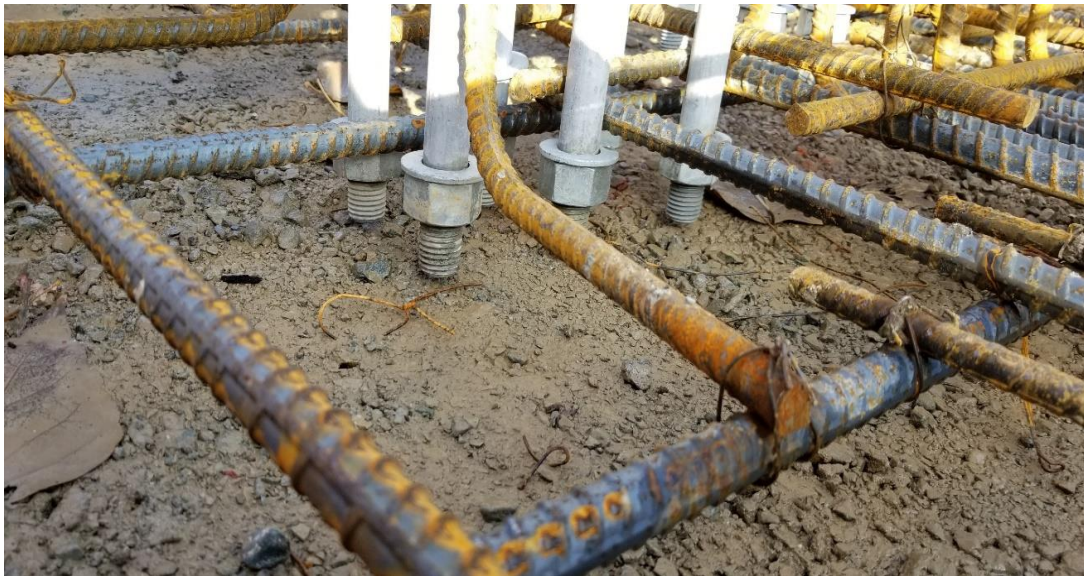
Reinforcing Steel and Structural Imbeds at Column Footings
