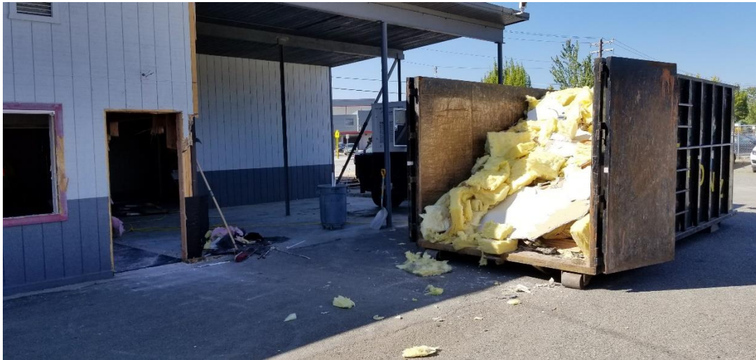
Demolition of the MTC
