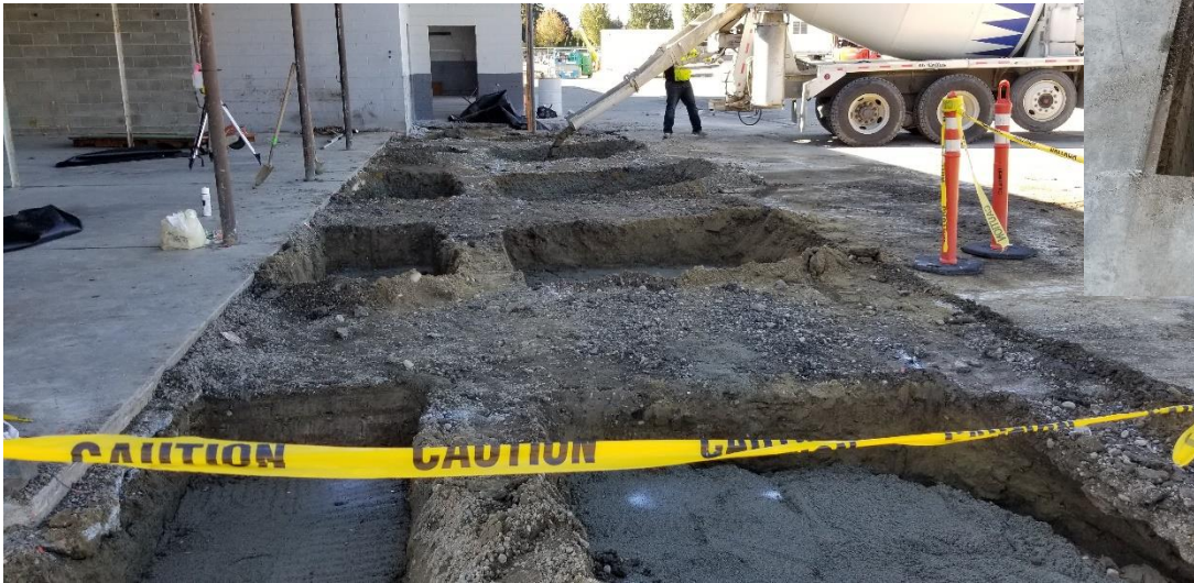
CDF Soil Excavation Reinforcement
