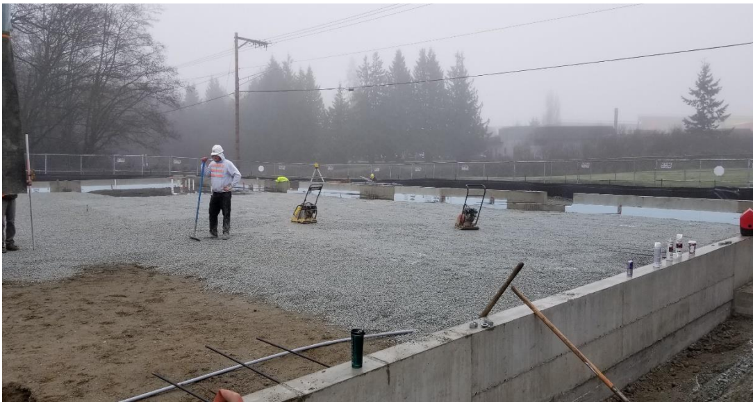
Underslab Gravel Subbase
