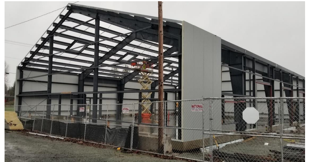
Installation of Insulated Wall Panels for Technology & Storage Building
