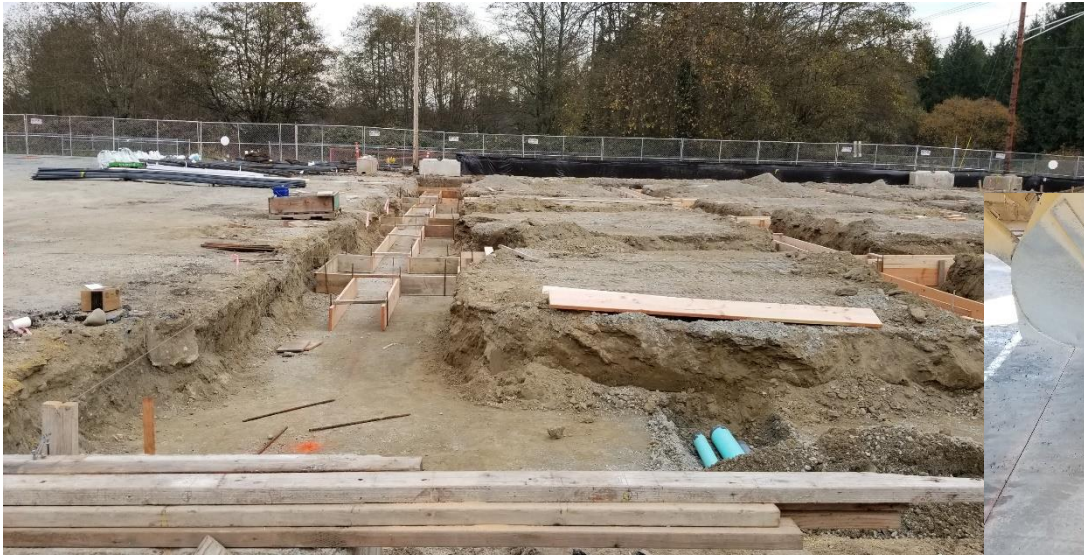
Footing Formwork for New Technology & Storage Building
