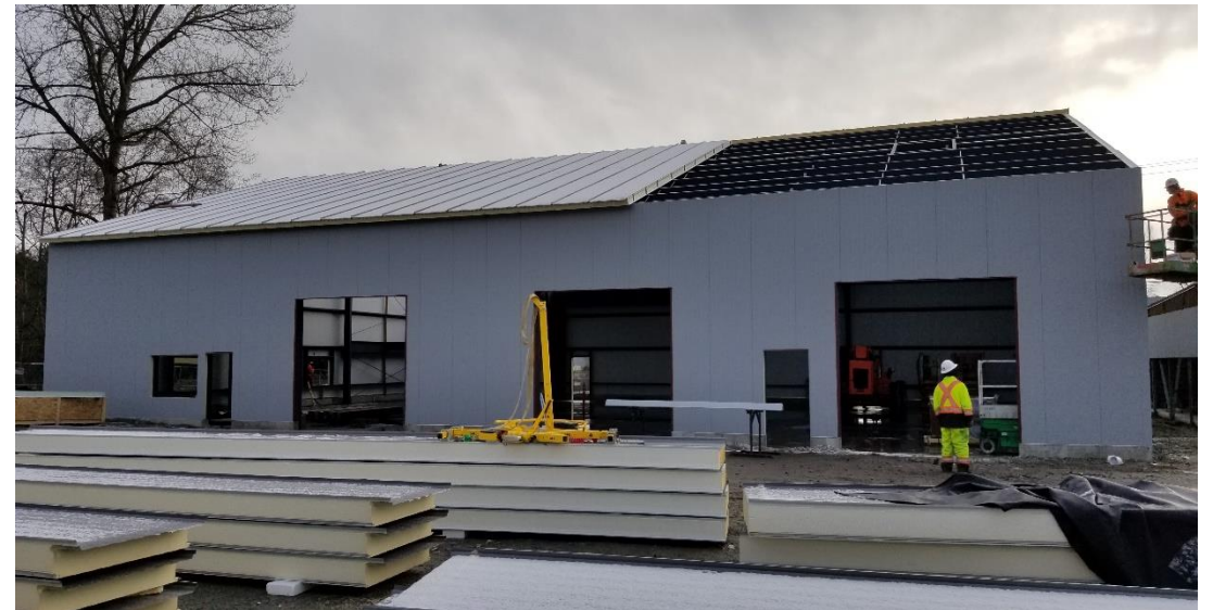
Installation of Insulated Wall & Ceiling Panels for Technology & Storage Building
